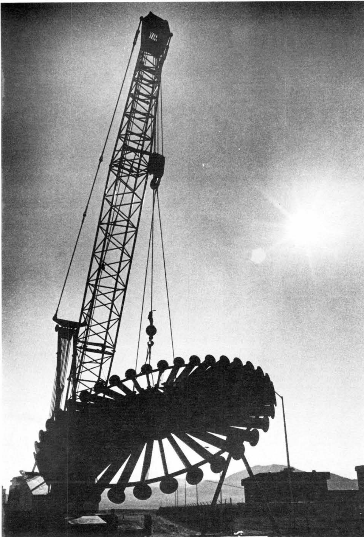
40-FT TRANSFORMER DAISY for Kirtland's child-care center? No, this is fusion art: A crane moved the innards of PBFA I into place at Tech Area IV where they are braving the natural elements — and becoming a new landmark for pilots taking off the runway.
